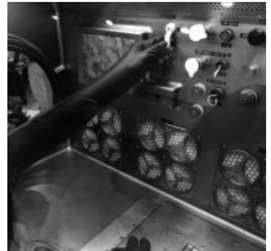
Figure 13. The MSG utility connections.
